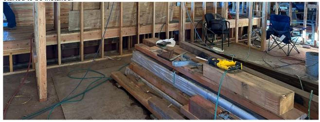
First Floor: most of the wall framing has been completed; electrical boxes and conduit is continuing to be installed; plumbing has started to be installed; material for fire sprinklers are on site and being stored in the Apparatus Bay; windows are on site and being stored in the Apparatus Bay.
