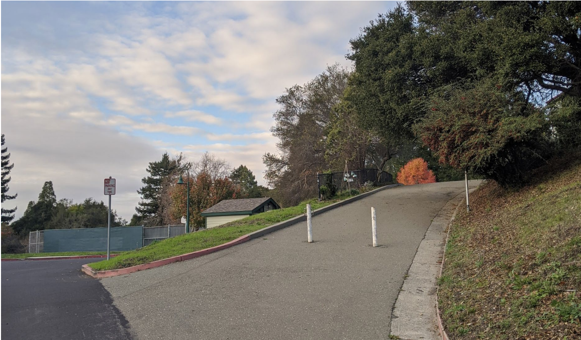
Figure 31: The connection between Windsor Avenue (darker pavement at left) and the Kensington Community Center.
