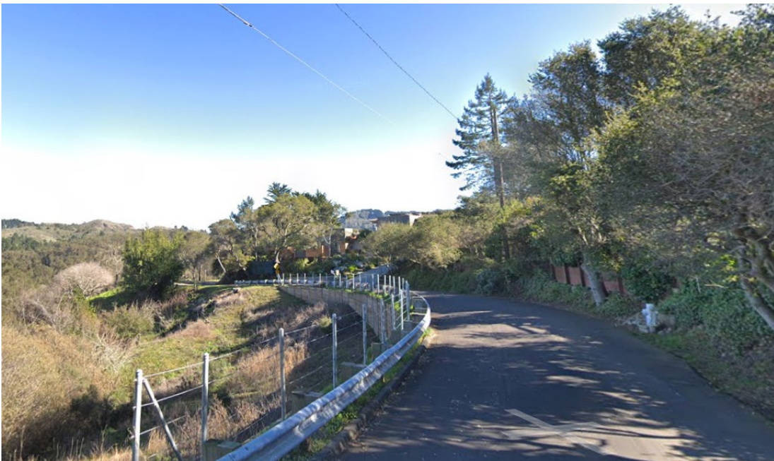
Figure 13: Los Altos Drive, looking east toward the sharp bend in which it becomes Beloit Avenue, taken from Google StreetView. This area along the retaining wall is only 17' curb to curb, despite the lack of any parked vehicles.
