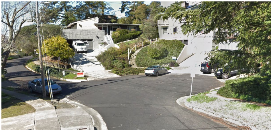
Figure 16: Vassar Avenue, looking north from the Alameda County line, taken from Google StreetView. This extra roadway could be particularly useful for passing/staging given the otherwise narrow (14-20') width of this segment.
